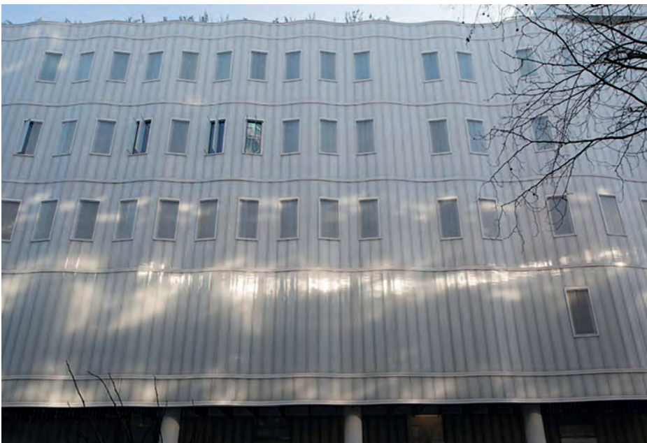
Left: The front façade of the Sainsbury Wellcome Centre has rippling glass panels representing waves of activity in the brain.
